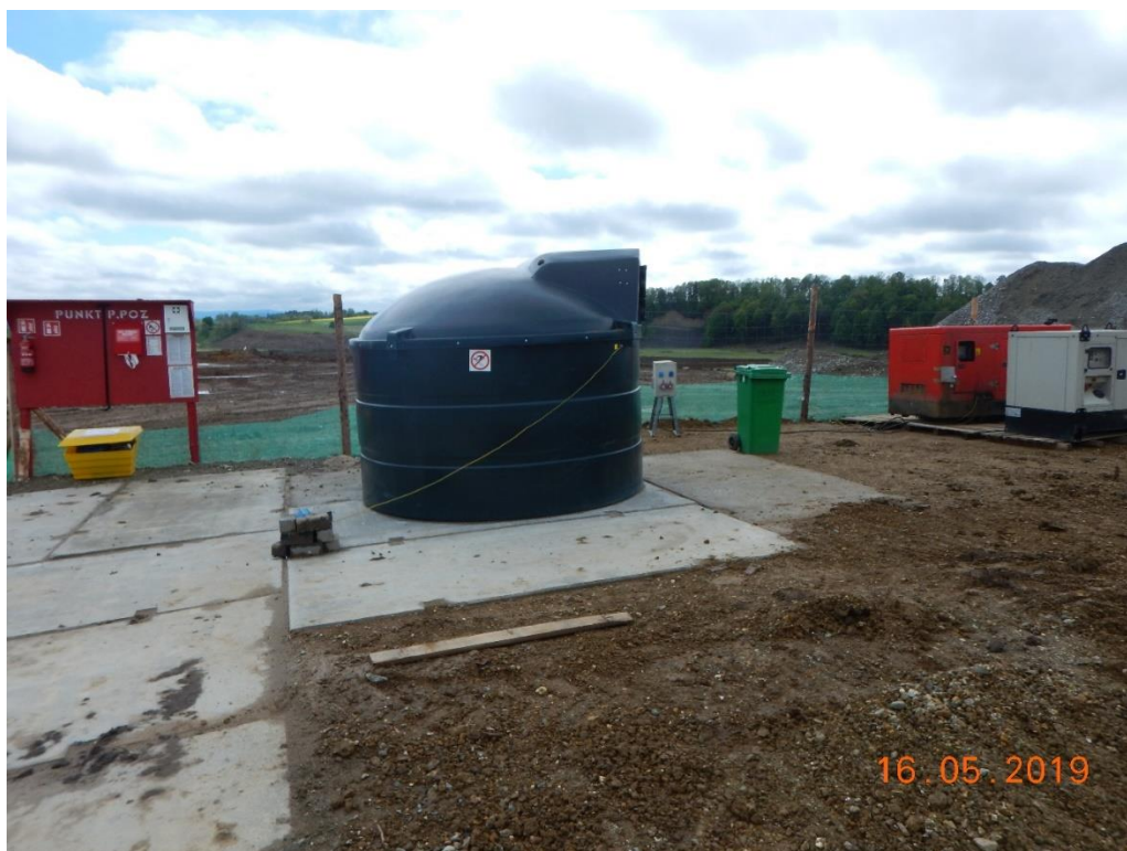
Phot. 2. Area for refuelling vehicles and machinery working on the site secured against spillage of petroleum-based substances to the soil (item no. 85 of EMP).
