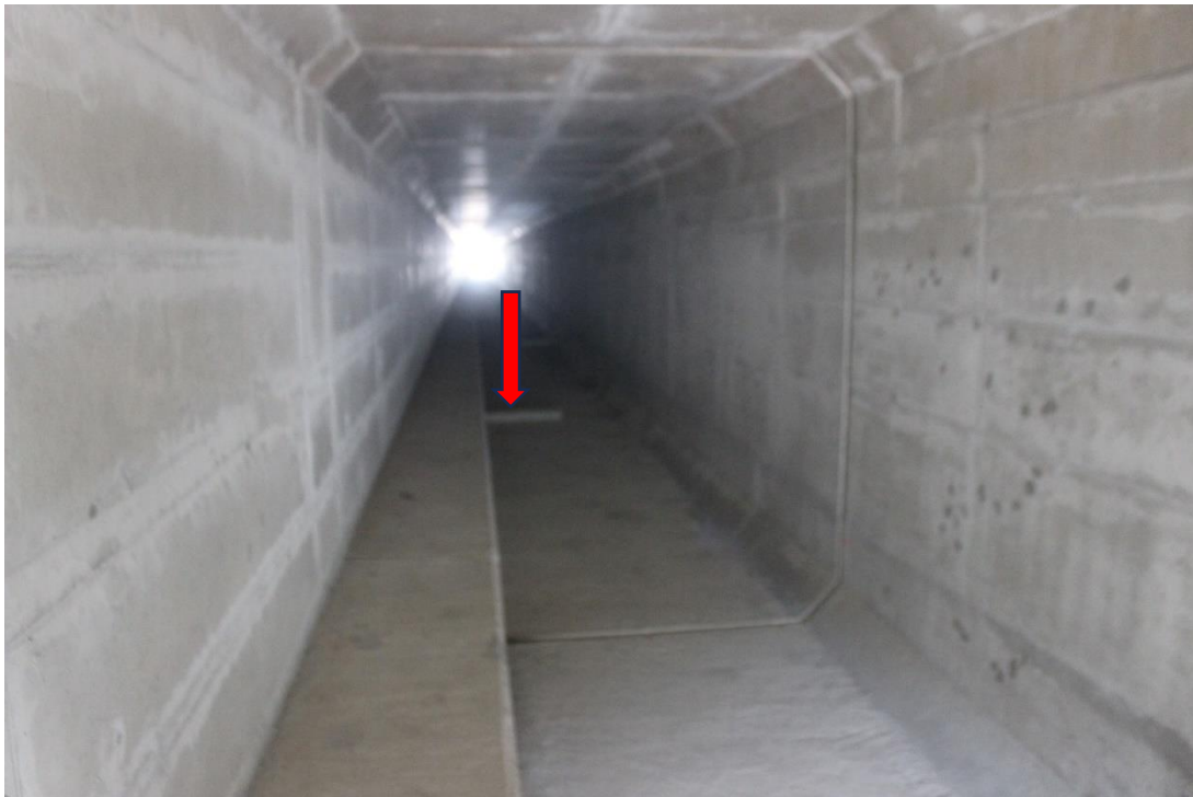
Phot. 12. Sills constructed in the sluice channel bottom – red arrow (item no. 56 of EMP).
