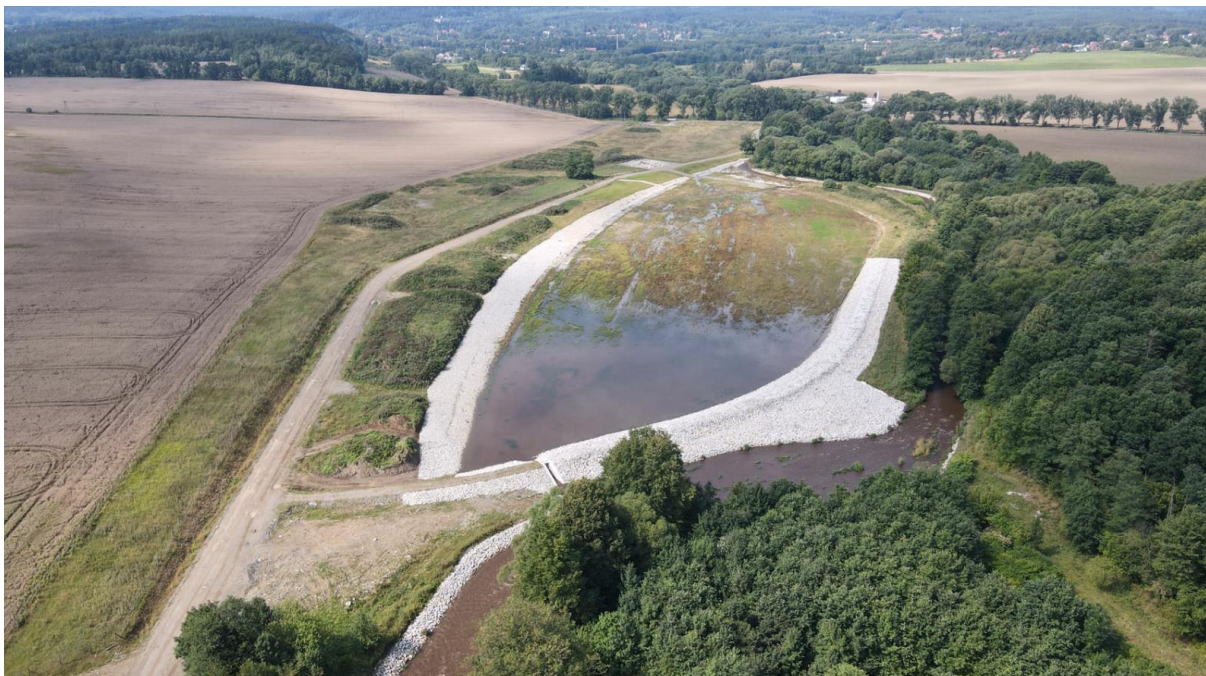
Phot. 17. Rubble trap constructed on the reservoir area.
