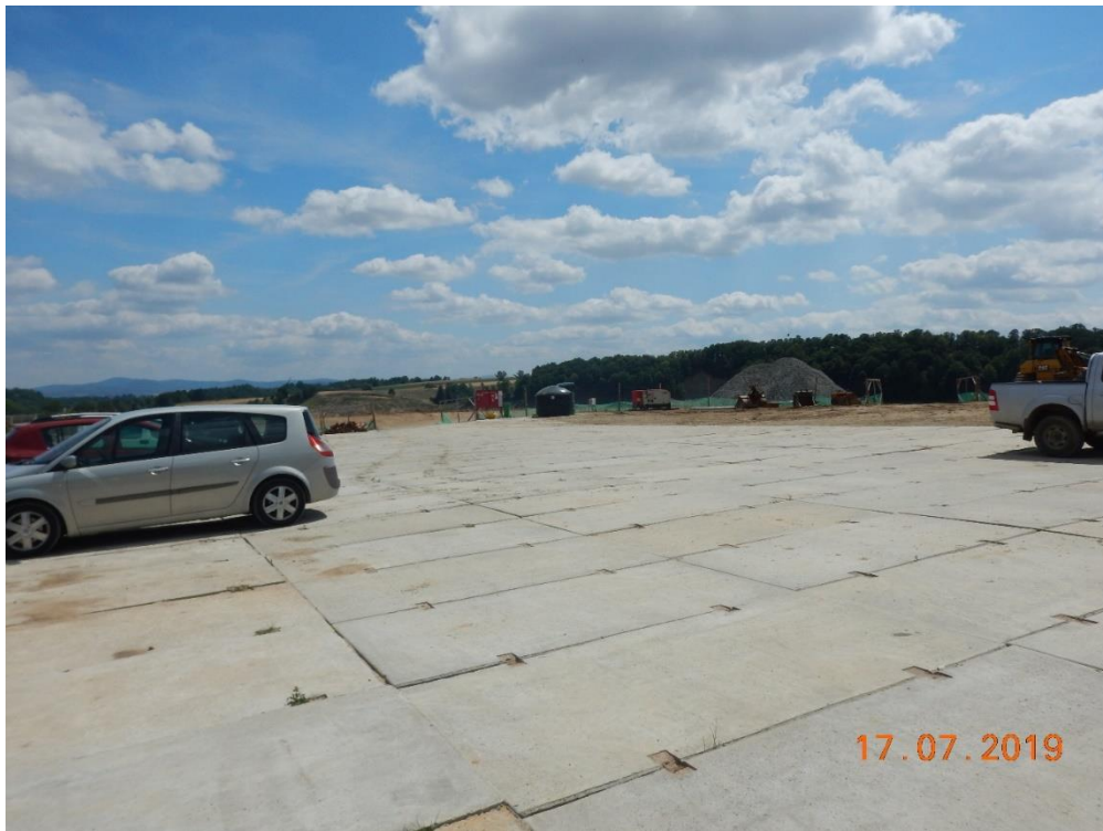
Phot. 1. Construction site facilities – site facilities' area was sealed from the ground (item no. 85 of EMP).
